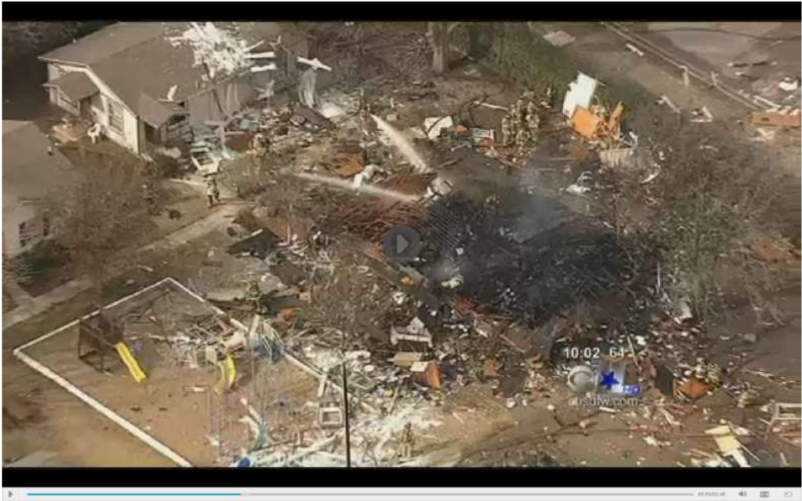
Natural Gas Distribution Explosion, Lewisville, TX - Jan. 2013
